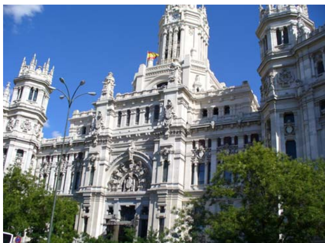
The new City Hall, Plaza de Cibeles
